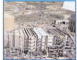
DAY FIVE All economizer tubes piped. AIG and ammonia system connected.
