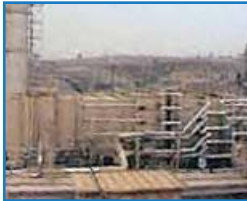
DAY ONE Existing System is shut down.
