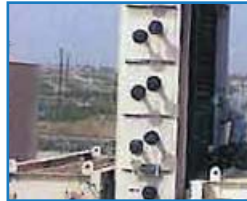
DAY THREE Slipping in the additional economizer.
