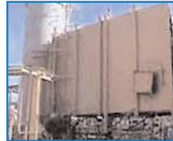
DAY FOUR Fitting transition duct to stack.
