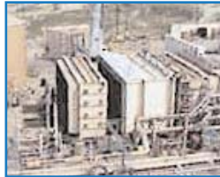
DAY TWO Stack moved 15 feet. SCR in place up against Economizer II. Rolling Economizer I to left.
